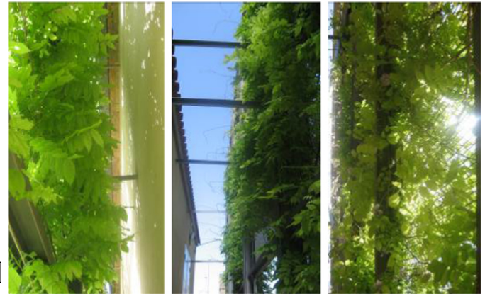
Fig. 2. Shadow factor in a double-skin green facade made with a steel modular trellis support and Glycine climber plants ( Wisteria sinensis ) [6].
