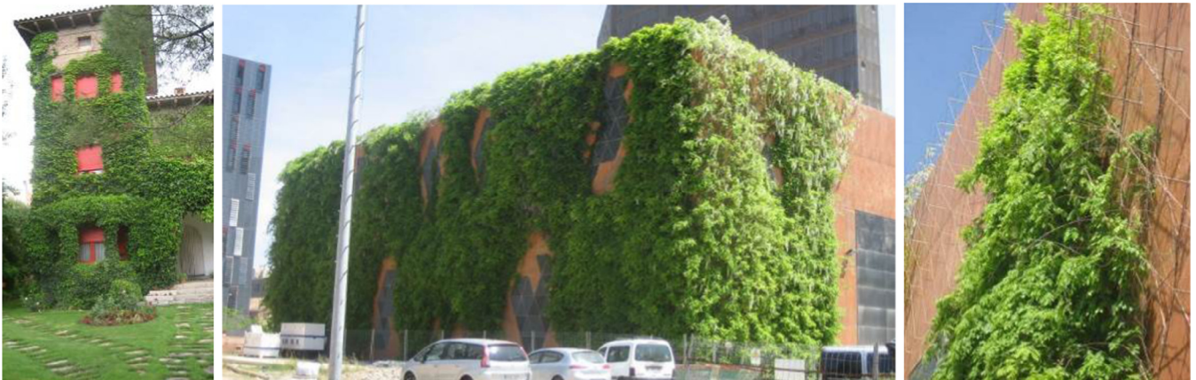
Fig. 1. Traditional green facade (left) versus double-skin green facade.
