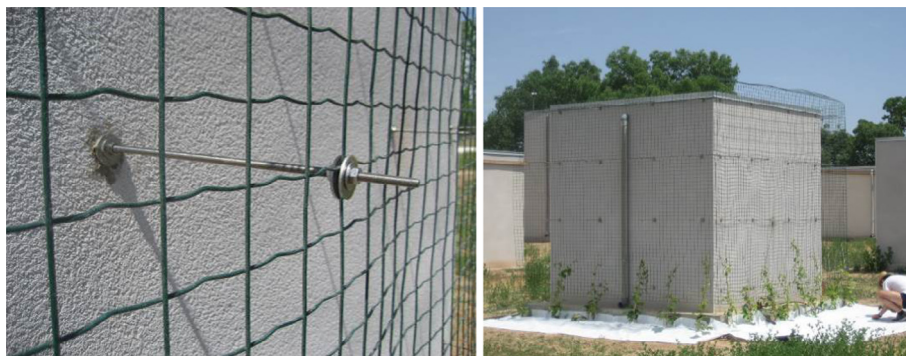
Fig. 5. Current double-skin facade. Constructive system details and general view.
